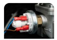
Low pressure switch at the gas inlet
